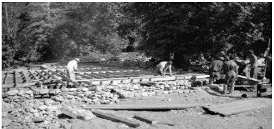
Big Sur Outdoor Theater Under Construction
