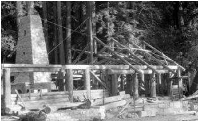
Big Basin Redwoods Lodge Under Construction
